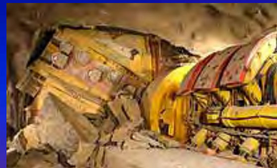
Tunnel Boring by Reaming - TBE
