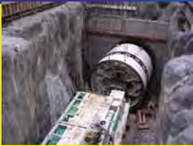
SMART Tunnel (Singapore)
