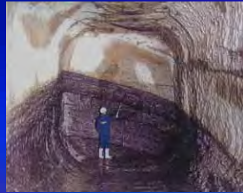
Non-Circular Section by Tunnel Boring Machine Technology
